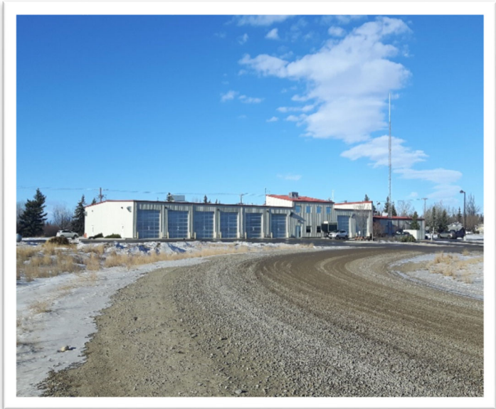
Looking northwest at the tri-services building
